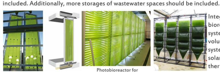
ntegration bioreactor to the wall system add more algae volumes and this wall system could act as shading and thermal insulation.
