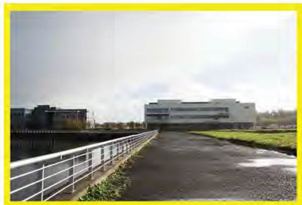
Fig. 21: The factors safety and maintenance are not met.
